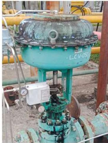
**Gambar 5. Level Control Valve 02-LCV-050**
