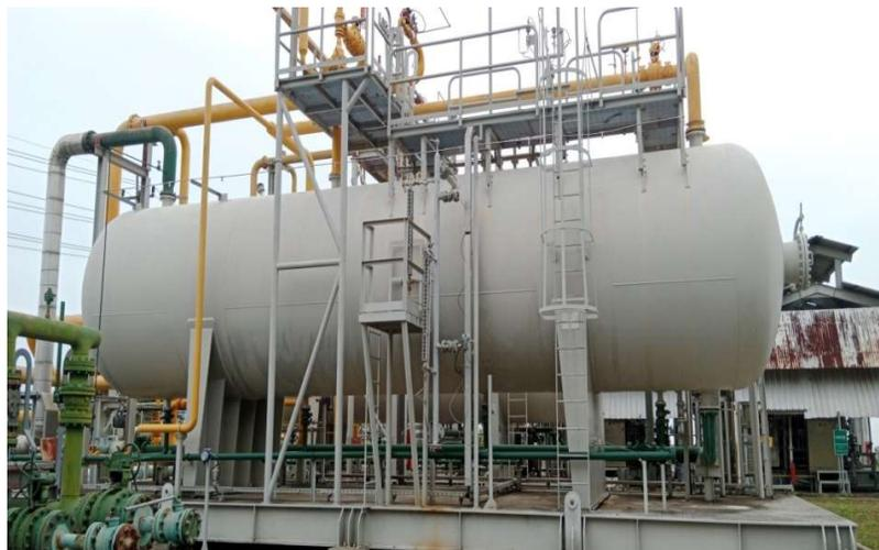
Gambar 2. *Production separator* di *Field Facility*
