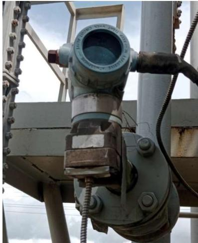
**Gambar 4.** *Level Transmitter 02-LT-050*
